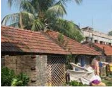
Brick walled tiled roof
