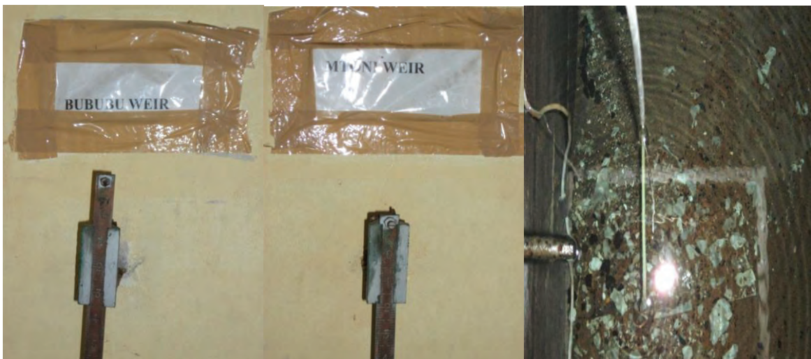
Plate 6-1 Bububu and Mtoni Water Gages and Measuring Chamber at Saatani Water Work Station
