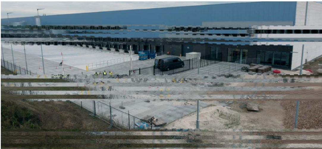
Figure 3.9 - example of interference on an industrial site.
