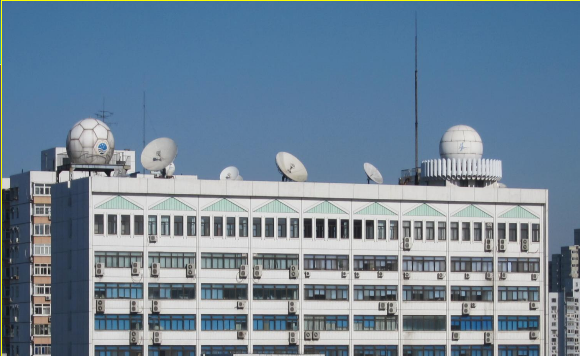
Beijing Ground station
