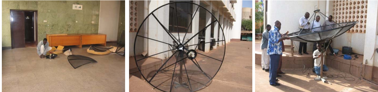
Figure 6: Assembling antenna, pointing and checking signal quality
