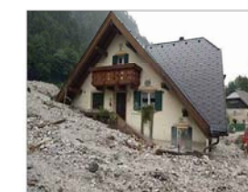
Damage from the 2003 debris flow event
