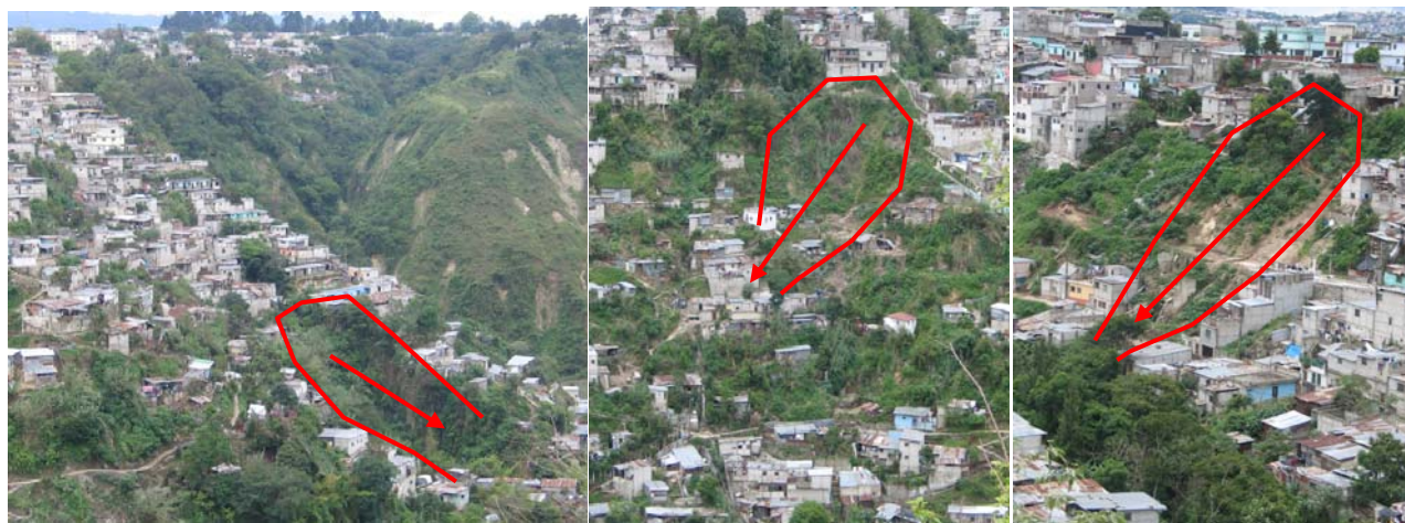
Figure: Typical examples of landslides that affect squatter areas constructed on steep slopes.
