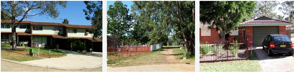
Fig. 1. Images of the Cranebrook estate, with the Neighbourhood Technology Centre on the right.
