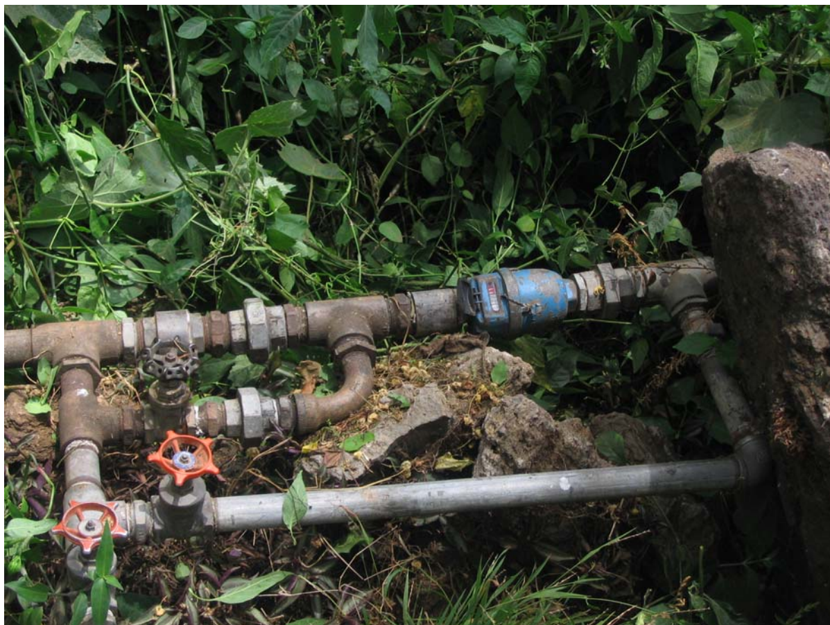
Figure 9. Illegal water abstraction through by-passing the water meter by a water user abstracting water from Lake Naivasha (photo: Hoekstra).
