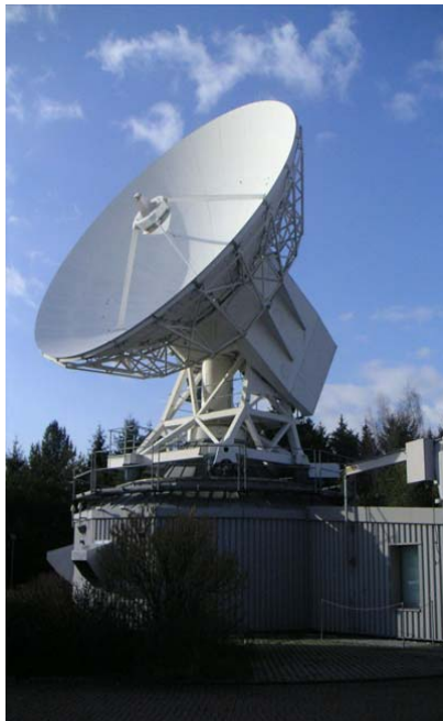
Meteosat Antenna Usingen, Germany
