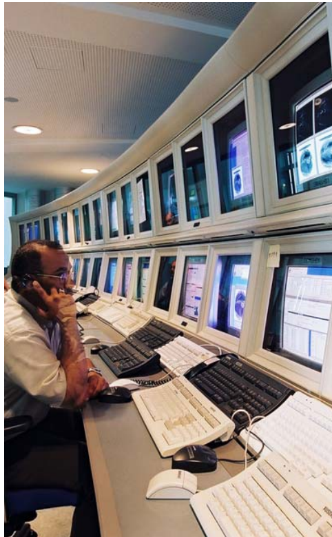
MTP Control Centre
